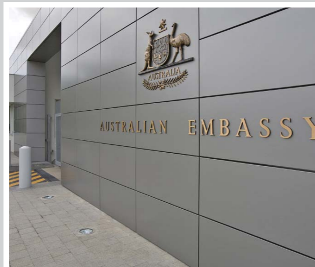
03 | Main Guard Booth, Australian Embassy in Phnom Penh
