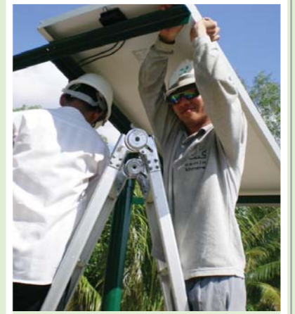
04 | Solar Panels Installations
